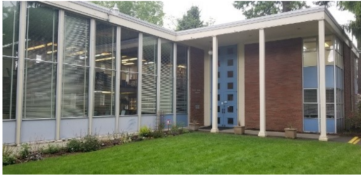
Cline-Tunnell Library at Western Seminary
